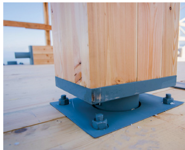
Custom steel connectors precision fit on-site
